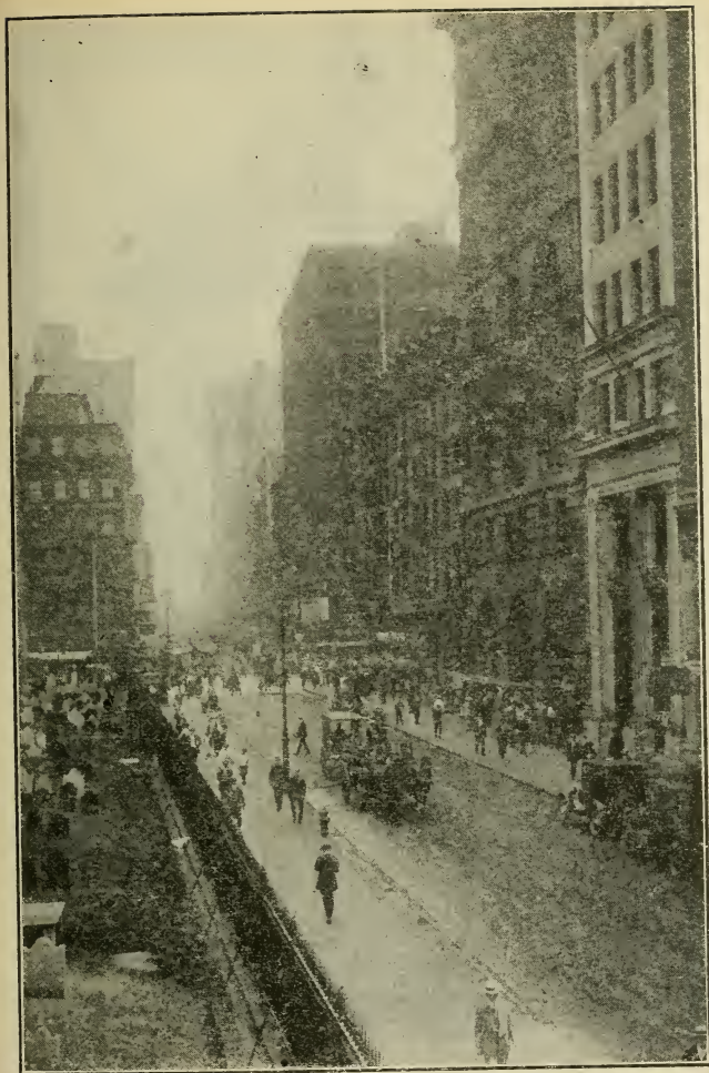
A view on Fulton Street, named after the inventor of the steamship. Looking east, St. Paul's churchyard on left.
